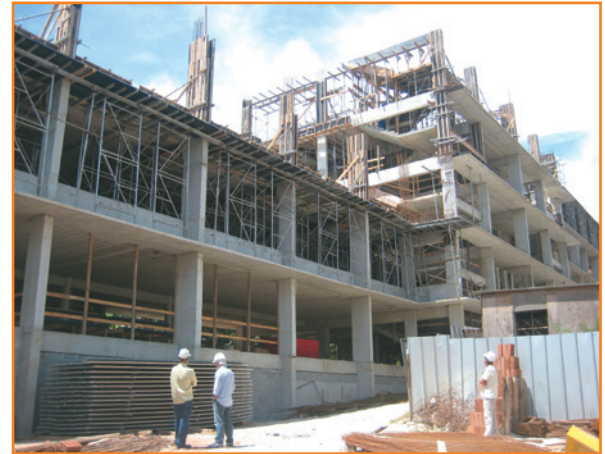
Figure 51 - Geoscience group headquarters at Federal Fluminense University, under construction.
